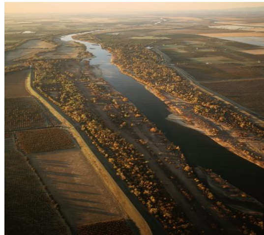
Agricultural levees built along the Feather River north of Sacramento, California. Photo by Michael Collier and courtesy of AGI.
